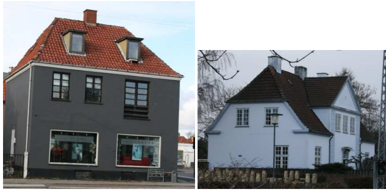
Figure 9 Two of the buildings in group D, both worth of preservation.
