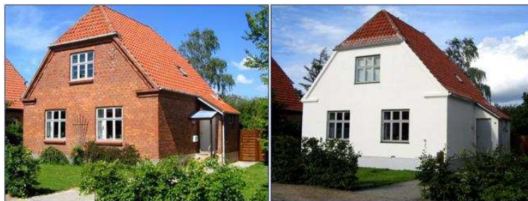
Figure 20 External re-insulation performed in practice (28).
