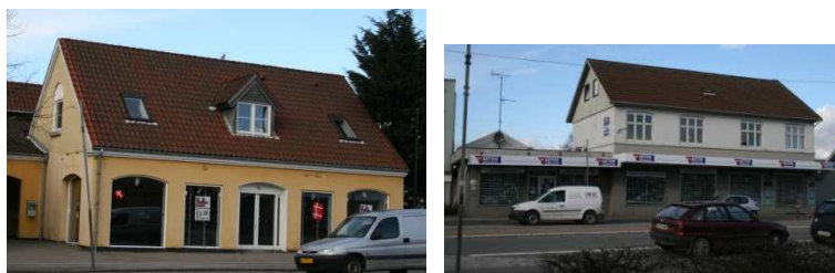
Figure 6 Examples of buildings for combined use from the period 1890-1929.
