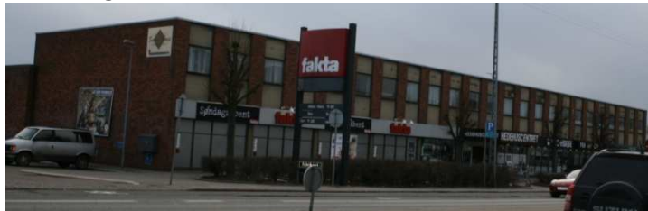
Figure 12 Hovedgaden 429, the centre, it is the only building in group H.
